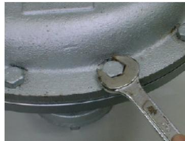
Action (22) : Attach spring ㉙ and spring plate ㉚. Secure spring chamber ㉛ with 6 hexagon head bolts ㉜.
